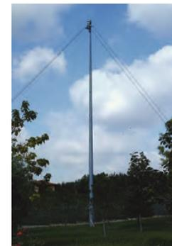
Delta antenna for HF communication in the ionospheric station of Rome, Italy
